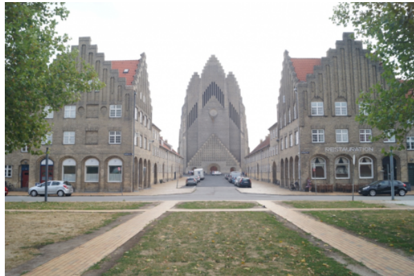
Peder Jensen-Klint (1853-1930), church dedicated to Nikolai Grundtvig, Copenhagen, 1921-1927. Built on the outskirts of Copenhagen, this church is part of an urban ensemble created by the same architect. Photo Simon Texier, 2018.
