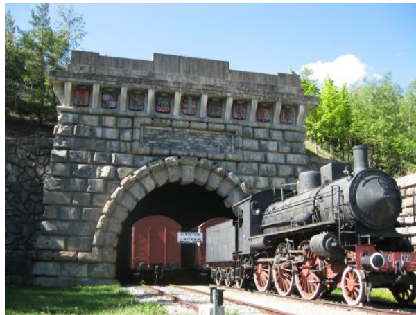
Monumental entrance to the Mont-Cenis tunnel, Modane, on the list of historic monuments since 1926.
