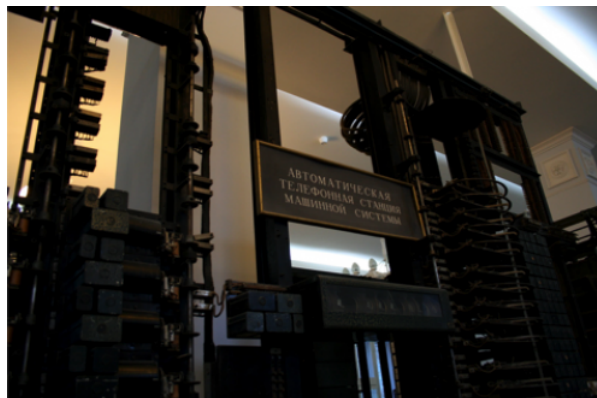
Soviet automatic telephone exchanges assembled at the Red Dawn (formerly Ericsson) factory as part of the technical assistance contract with Ericsson (late 1920s). Moscow Polytechnic Museum. Photo credits : Grégory Dufaud.
