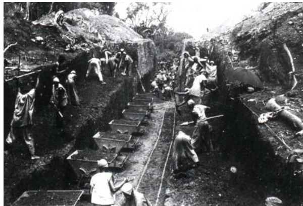
Building of a railway in Dahomey around 1900. Photo: Roger Viollet
