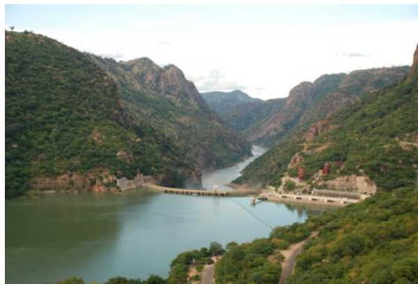
Le barrage de Cabora-Bassa, au Mozambique. Source : Climate and development knowledge network .
