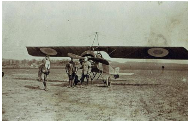
Monoplane Morane-Saulnier, « parasol », type L (1913), whose rotary engine Gnome 80 CV was a model for the German aeroplane “German Taube”. Source : www.britmodeller.com
