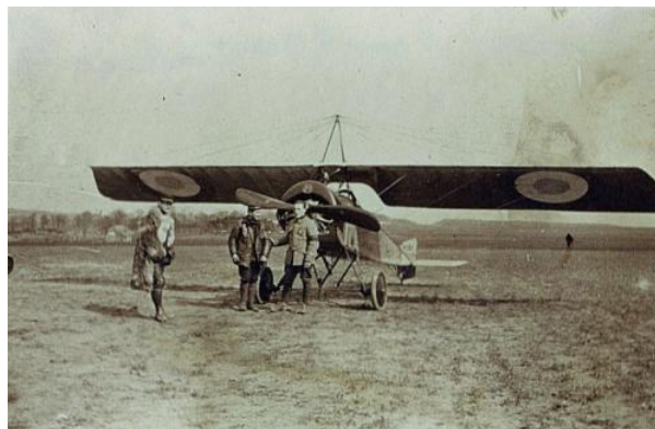
Monoplane Morane-Saulnier, « parasol », type L (1913), whose rotary engine Gnome 80 CV was a model for the German aeroplane “German Taube”. Source : www.britmodeller.com
