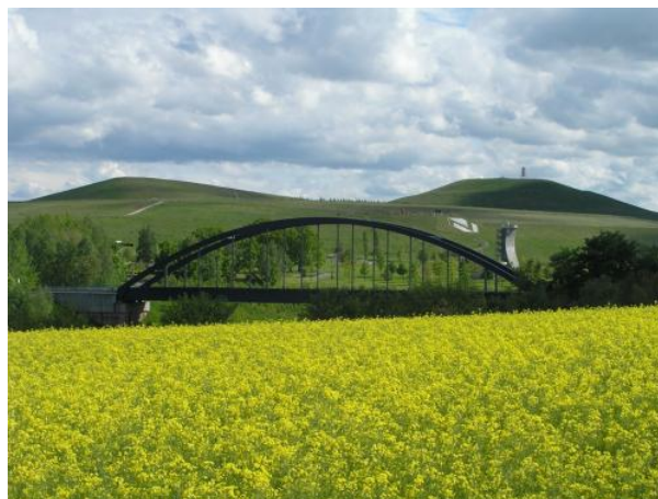
Illustration 4: Ronneburg's new landscape (photo Deshaies, May 2013). A butte composed of slagheap rubble used to fill in the excavation now stands at the site of the former open-pit uranium mine. Hardly any visible traces of former
