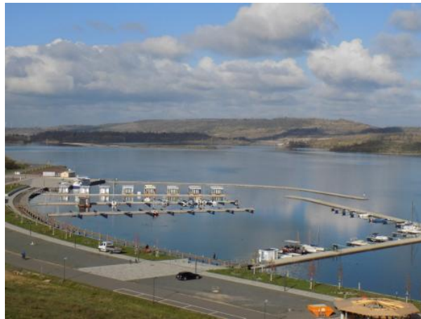
Illustration 3: The former lignite mine in Geiseltal, south of Halle in Saxe-Anhalt (photo Deshaies, October 2019). After operations stopped, in 1994, at one the largest lignite mines in Germany, residual excavation was submerged by a lake that spreads over a surface of 1,900 ha. (4,700 acres) to a maximum depth of 78 m. (256 feet). In 2011, after the lake's level had settled, two marinas, like the one shown here, were established.
